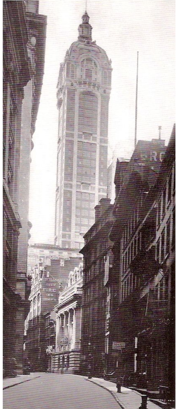
The Singer Building towers over its neighbors in this 1908 photograph taken from a nearby New York Street corner
